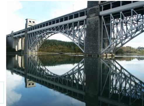
Two-tier steel truss arch bridge
