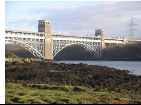
Two-tier steel truss arch bridge
